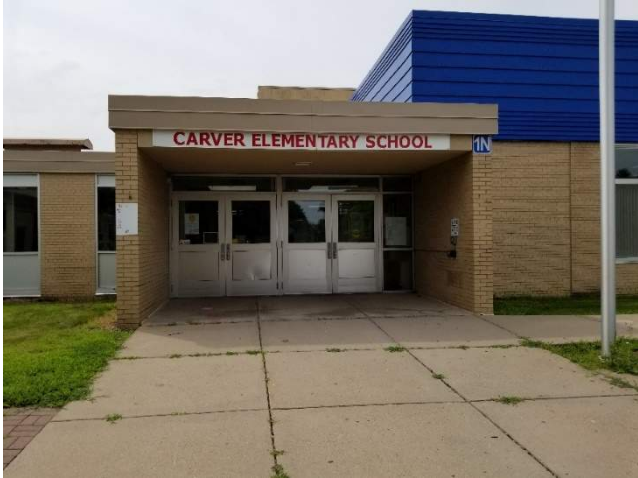
A building-mounted sign was mounted on a portion of the building that was removed as part of an earlier phase of construction – approximately 9 SF
