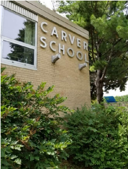
A building-mounted sign was mounted on a portion of the building that was removed as part of an earlier phase of construction – approximately 38 SF
